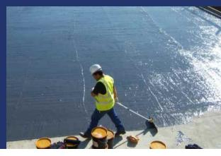
INDOSIT<sup>™</sup>WP 2002 is high performance water proofer that dries to form a tough impermeable coating. It is a blend of tropical grade bitumen emulsion with 8% added pure acrylic polymer.
