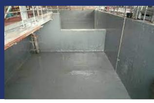
INDOSIT <sup>™</sup> WP 1003 is a pre – packed two component polymer modified cementitious coating, which can be easily mixed on site and applied with brush or roller. This coating cures to form elastomeric waterproofing membrane with excellent adhesion to cementitious surfaces.
