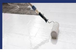
INDOSIT<sup>™</sup> PU 2003 is a premium, liquid applied, highly permanent elastic cold applied and cold curing, one component polyurethane hybrid membrane used for long-lasting water proofing
