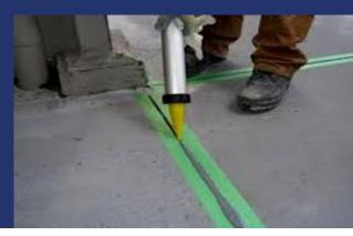
INDOSIT <sup>™</sup> PS 5001 is two packs Polysulphide based, tough flexible durable with strong adhesive sealant basically used for movement joints in concrete and pavements. When the two packs are mixed and it forms tough, flexible durable rubber like material with strong adhesive property on most building substrates and joints.
