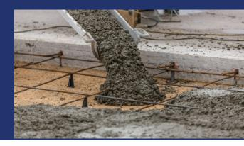
INDOSIT<sup>™</sup>LP 9001 is a new generation superplasticiser based on polycarboxylate ether. It is developed to achieve high early strengths for all grades of concrete where high early strength and performance is required. INDOSIT<sup>™</sup>LP 9001 is compatible with all Portland cements meeting recognized international standards and is free from chlorides and has been formulated to comply with ASTM 0494 for Types A and F admixtures
