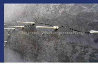
INDOSIT<sup>™</sup> GA 3015 is an expanding crystal modified high strength grout admixture for pressure/injection grouting. By introducing into the concrete mix, wet volume expansion and increased fluidity along with enhanced bonding, without segregation are produced.
