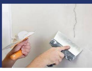
INDOSIT $^{\text{TM}}$  CF 3011 is a cement based polymer modified powder material for filling cracks in plastered surfaces. It is ideal to fill 2 to 3 mm wider static cracks, it has strong adhesion and also non-shrink in nature.
