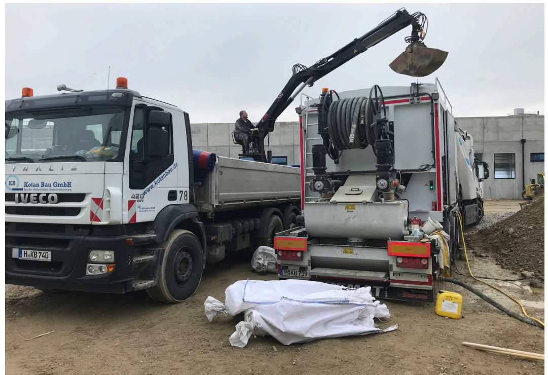
Loading the pump-truck with VELOSIT SC 252 and sand
